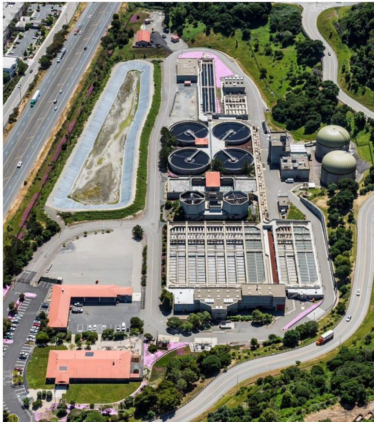
(Clockwise upper left to right): Effluent Storage Pond, Maintenance Annex (red roof behind the pond), Chlorination/Dechlorination Building, Chlorine Contact Tanks, Effluent Pump Station, Secondary Clarifiers, Organic Waste Receiving Facility, Solids Handling and Cogeneration Building, Digesters and Digester Building, Aeration Tanks, Biotowers, Primary Clarifiers and Blending Channel, and Headworks. The two orange-roofed buildings in the lower left are the Maintenance Building (top) and the Administration Building (bottom).
