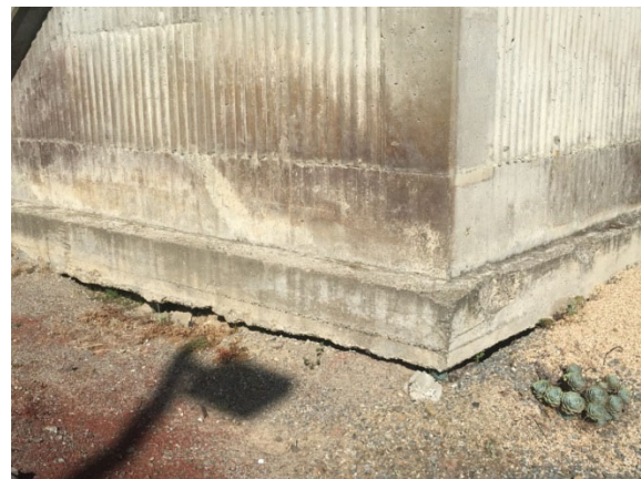
Exposed bottom of process tank
