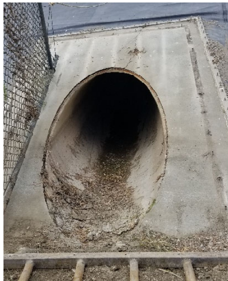
Pond Inlet and Headwall
