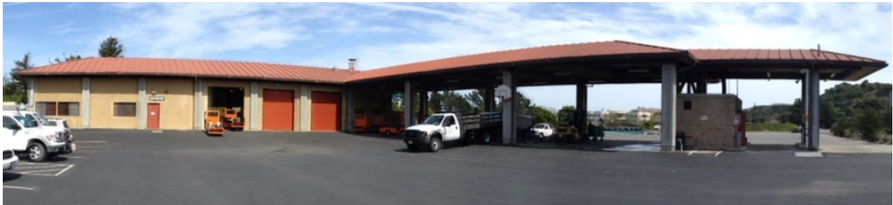
Maintenance Building with standing seam metal roofs
