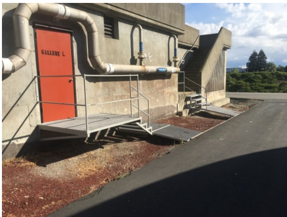
Stair modifications to account for settlement
