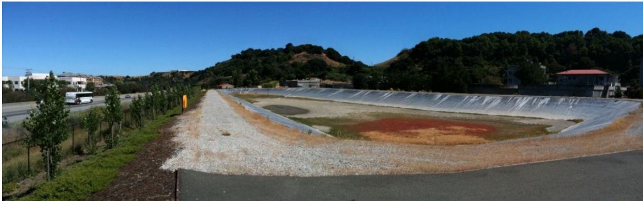
Effluent Storage Pond
